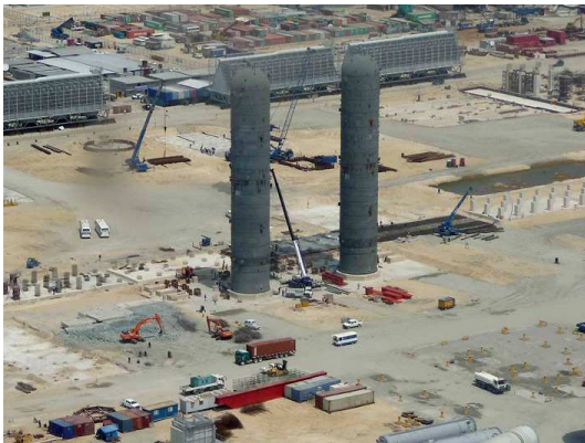
Escravos Gas-to-Liquids, Nigeria Foto: Bilfinger Berger
